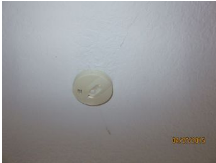
Replace old smoke detectors
