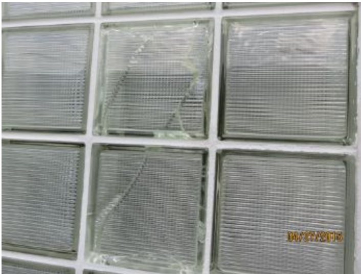
Broken glass blocks on east side on house
