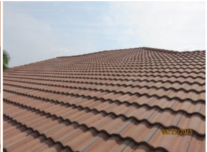
View of roof covering
