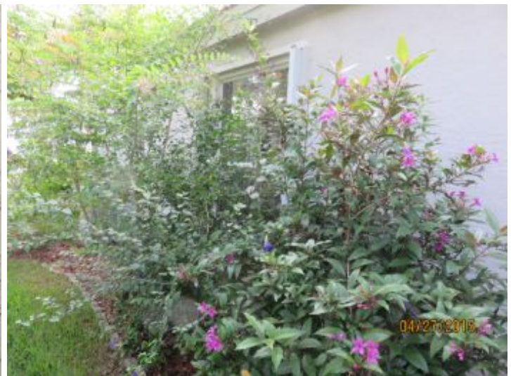
Cut trees and shrubs from exterior and roof
