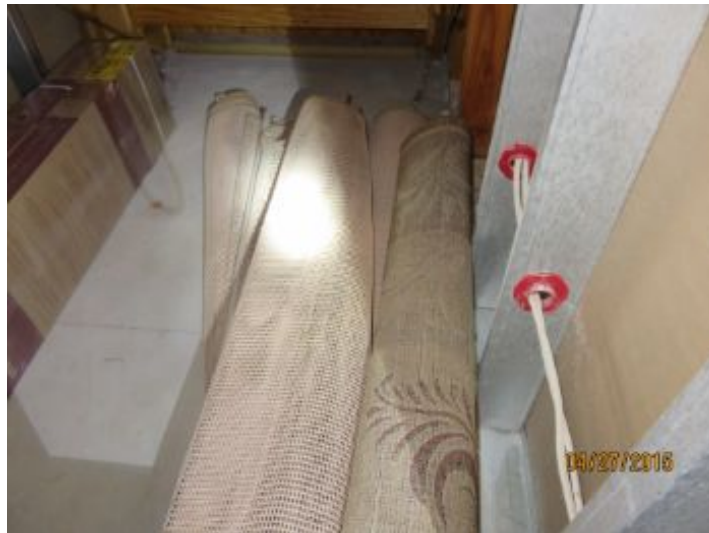
Pool fence under stairs
