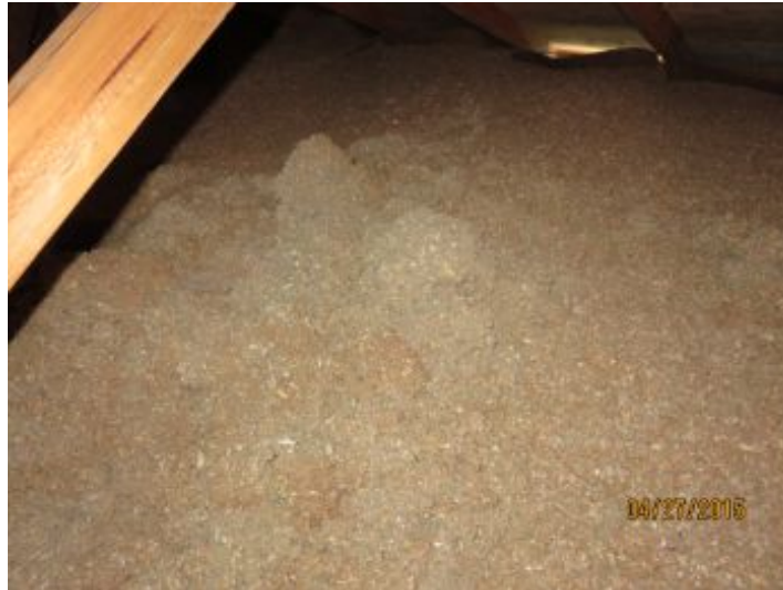
Loose fill insulation in attic
