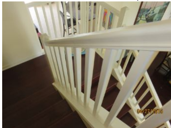
Check railings for safety on regular basis
