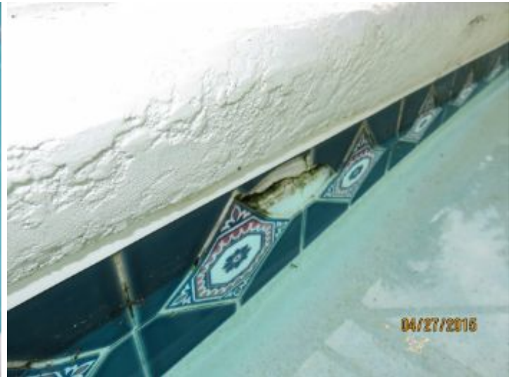
Cracked/broken tiles
